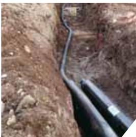
Reused for backfilling
